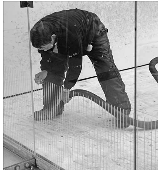
Repairs are underway at the 17 Wing squash courts. Photo: Bruce Tulloch
