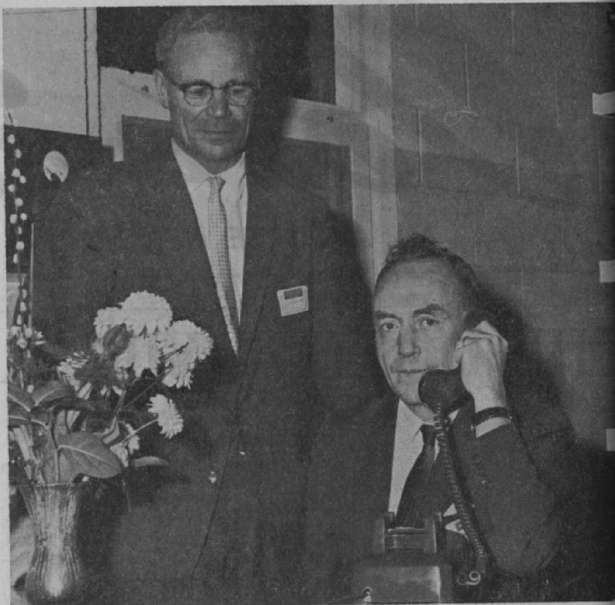
FIRST CALL: The first long distance call from the new Gimli dial exchange was placed April 21 by Group Captain G. Sutherland, Commanding Officer of the RCAF Station near Gimli. Standing is Construction Superintendent C. T. Woodman, of The Manitoba Telephone System.
