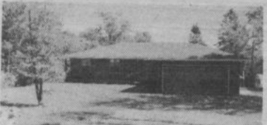
LAKE ECHO $115,000: Very deceiving bungalow. SUPER SPACIOUS. Main floor family room with fireplace. Double garage.
