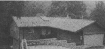
NO SMOKING HOME: Large sundecks. Immaculate, private setting backing onto Mill Hill Park. $134,500.
