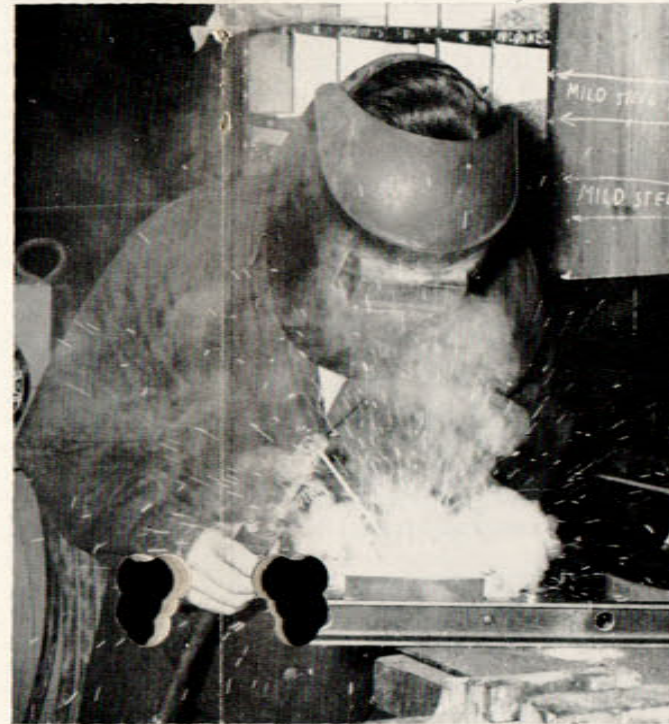
The "Man in the Iron Mask" is Cpl. "Thorny" Thornhill. He is arc welding fire extinguisher brackets.
