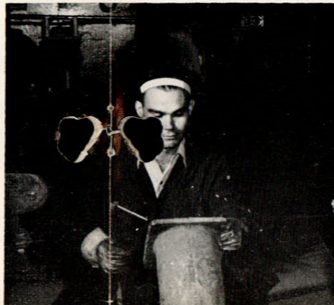
Thorny checks his weld on steampipe fittings.
