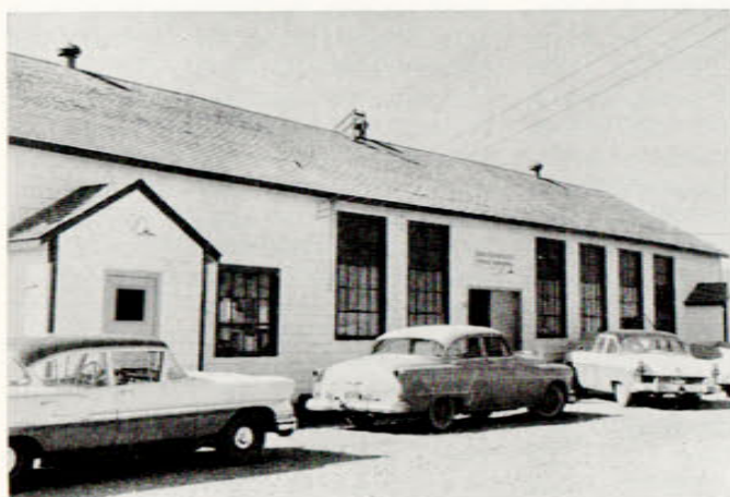
Exterior view of the Station Hobby Shop.
